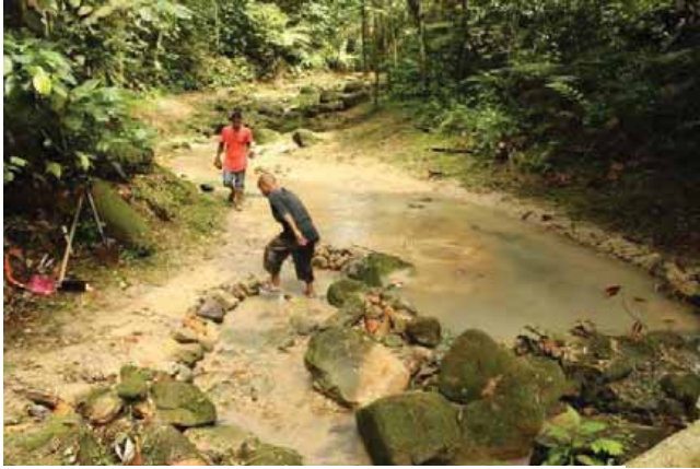
Stabilising the banks with rocks
