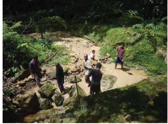
Removing excess sand
