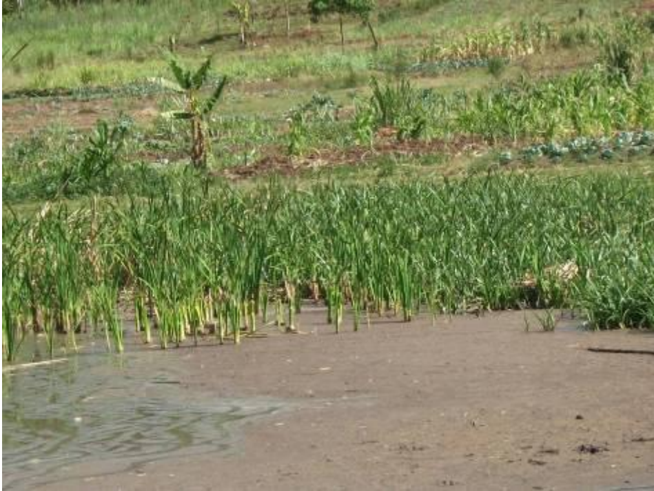
A section of the dam where water is drying up at an Alarming rate.
