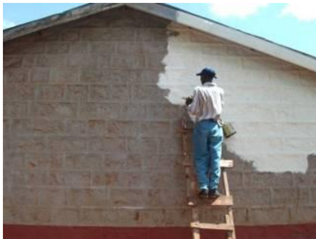
Artist Maina preparing the wall with undercoat paint
