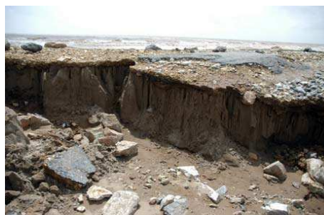
Dyke eroded severely due to not being protected by mangrove forests (Photo: Pham Hai, Vietnamnet, 28/9/2005)
