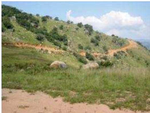
Figure 8: New road construction leading to erosion
