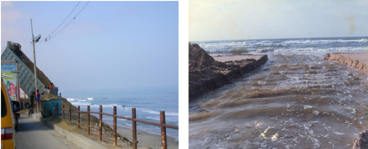
Figure 16: Sewage discharge into sea (Wadi Gaza).
