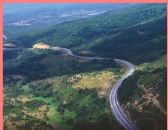
Figure 128. Regional road Bitola-Resen is breaking bio-corridor of Brown Bear (fragmentation of habitats) (Photo: M. Dzingo)
