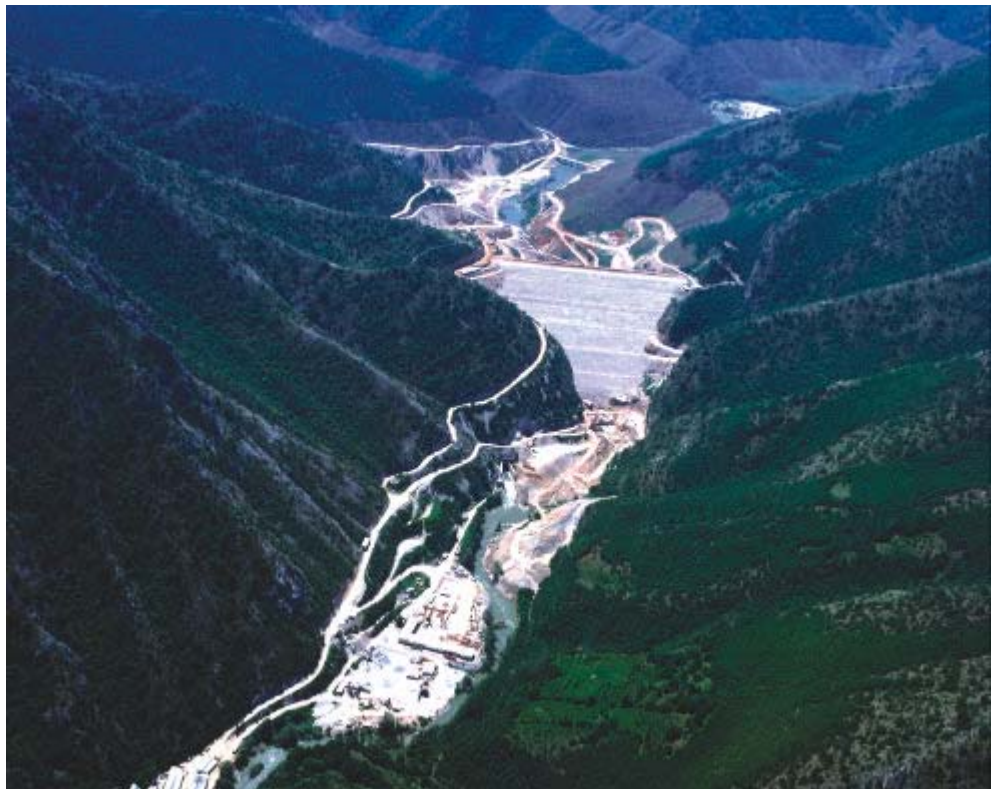
Figure 121. Kozyak Dam (in construction) (Photo: M. Dzingo)
