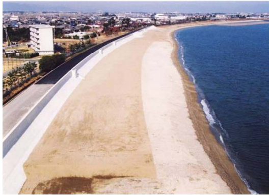
Restoration of sandy beach (Sand from nearby areas was used in consideration of the ecosystem)
