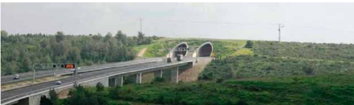
Monitoring programs that are conducted at each of these locations have shown heavy usage of these overpasses by wildlife. Photos: Dotan Rotem, NPA
