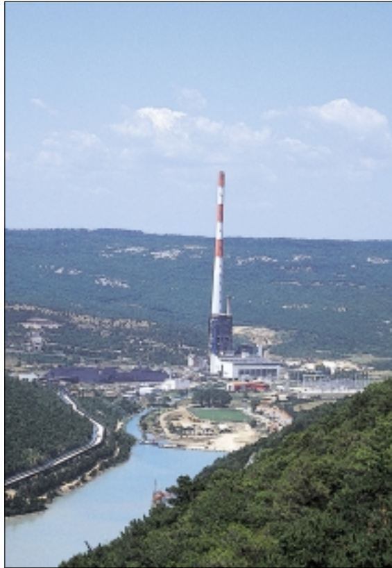
Figure 77. Thermal power plant Plomin in Istria
