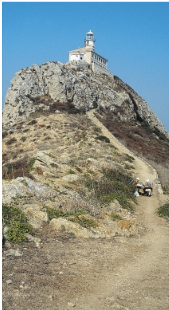
Figure 66. Lighthouse on the island of Palagruža (photo by D. Grlica)
