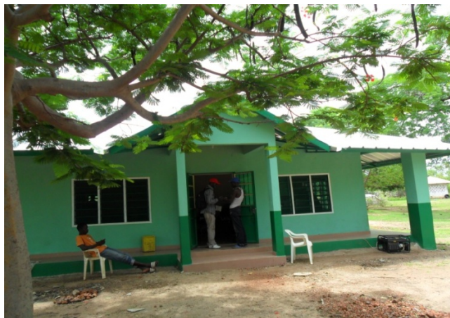
Fig 13: newly built office block in Dumbuto Camp
