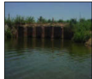
Picture (7-27) Hawis (to control water flow)
