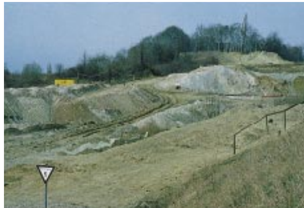
Construction of the B 42 Motorway, Kuckstein, Siebengebirge
