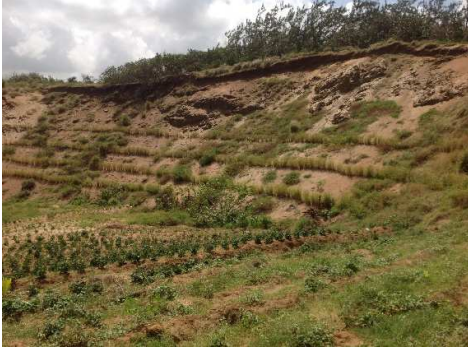
Photograph shows planting of Khus Khus grass and food crops on the slopes of an excavated sand dune at Walker's Reserve
