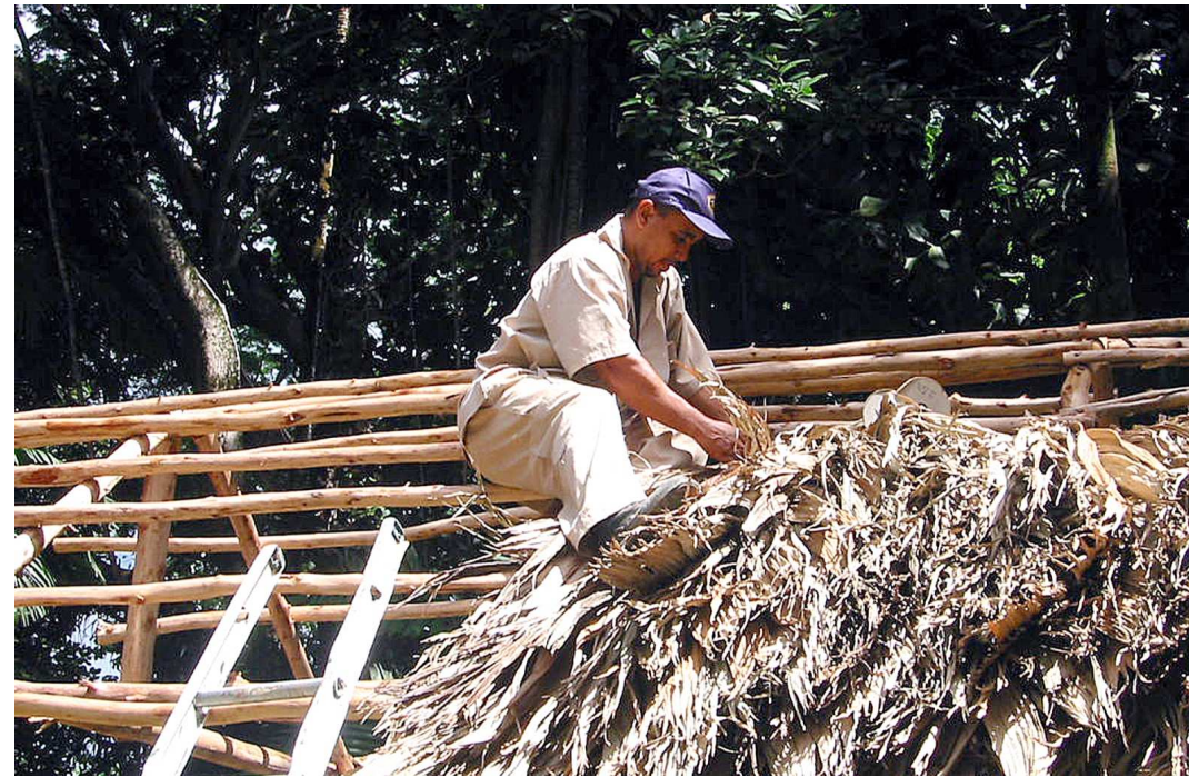
'Latannien fey' has traditionally been used for thatching. Harvest is currently probably sustainable, but what about the harvest of coco de mer?
