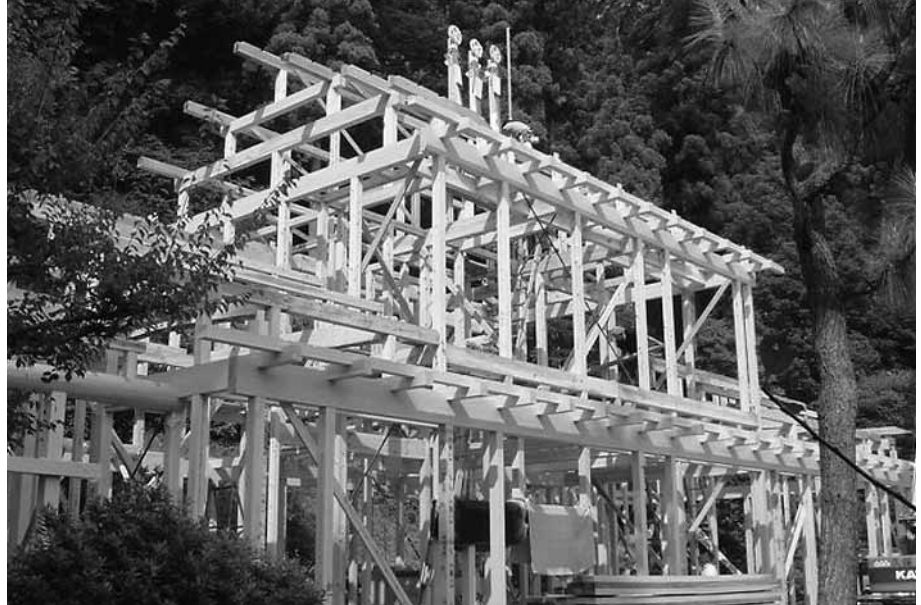
Building a house with Tokyo timbers - the framework completed
