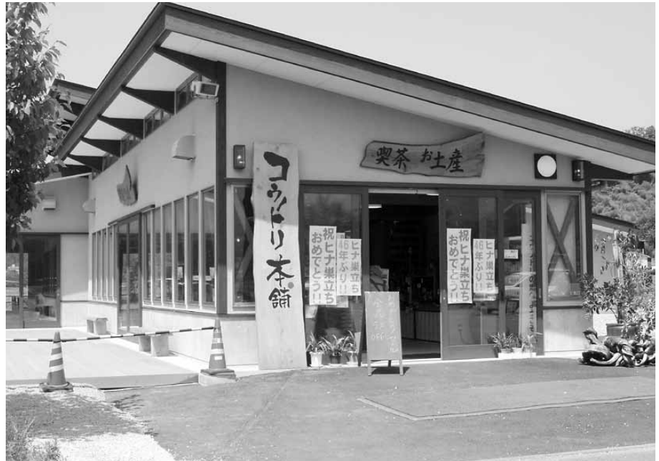
Local communication center "Konotori Hongo (Oriental White Stork Shop)" run by Toyooka City
