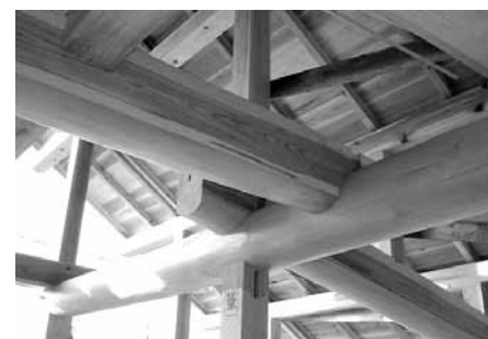
Wooden frames under the roof
