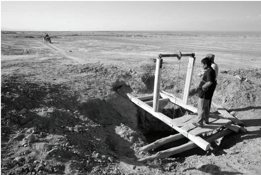
Figure 4. Digging a vertical shaft (photo courtesy of Geroge Steinmetz).
