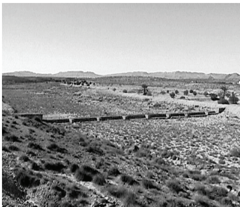
Figure 7. Gabion unit on Wadi Naguab.
