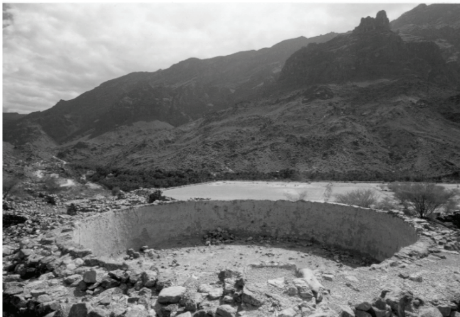
Figure 5. Liggil water tank for water distribution.
